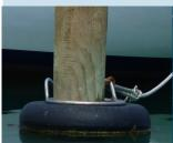
This image shows the correct way to attach your mooring lines to a floating ring.
