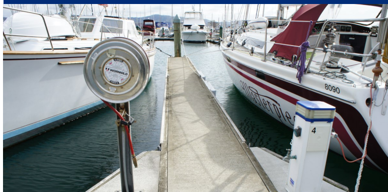
Please use the marina fire hoses in an emergency only
