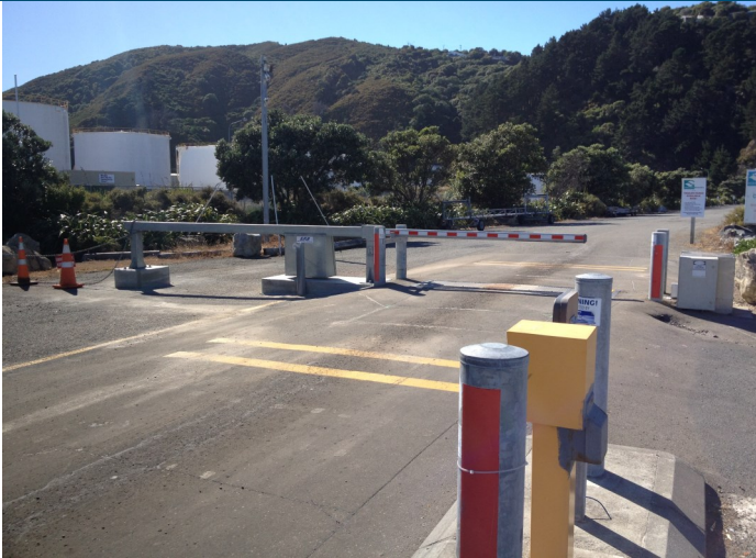
The old barrier at the entrance to the launching ramp has been replaced with a new sliding arm.
